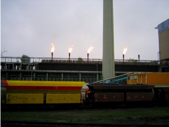
Smokeless bleeder system in operation
